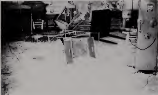
Damaged equipment in Cafeteria kitchen
