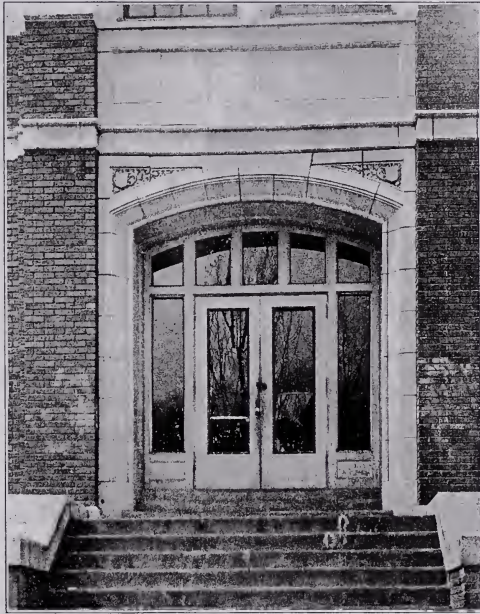
MAIN ENTRANCE ON FOURTH STREET
